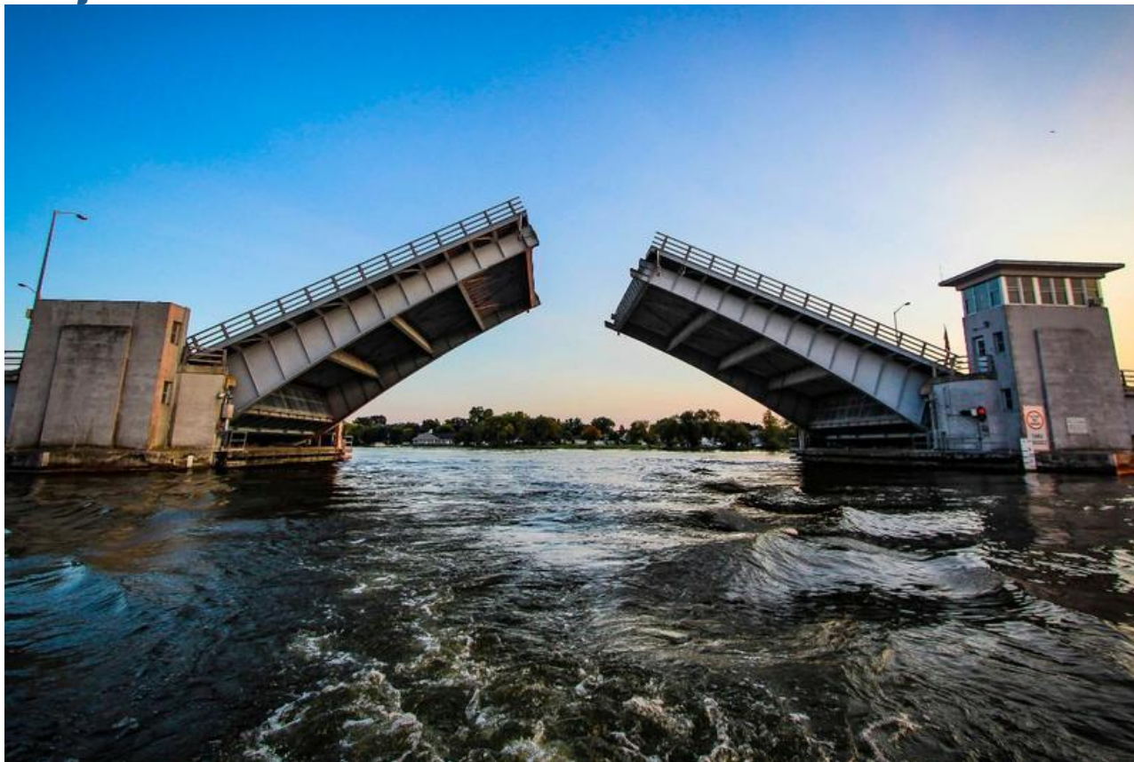
Oshkosh Avenue (WIS 21), city of Oshkosh, Fox River Bridge
