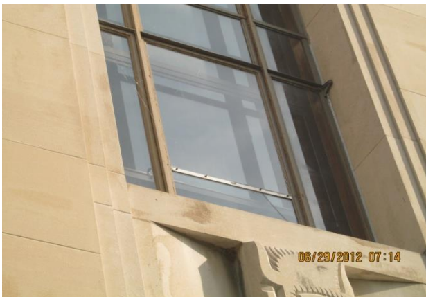
Deteriorated window framing replaced
