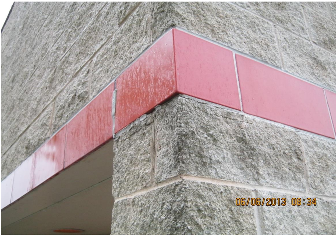
Highway Shop failed mortar joints
