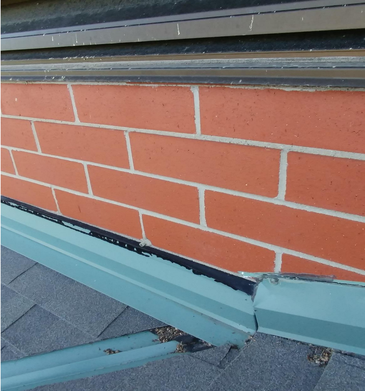
Damaged and deteriorated flashing joints
