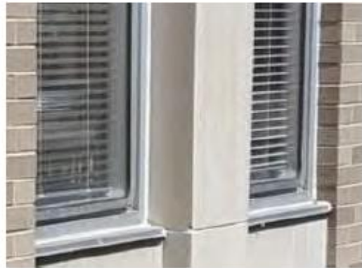
Illustration #1: Illustrates sealant failure and limestone in need of cleaning
