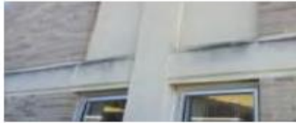
Illustration #1: Illustrates sealant failure and limestone in need of cleaning
