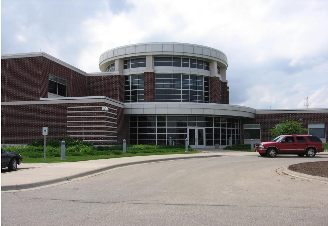
Front lobby window system to be replaced
