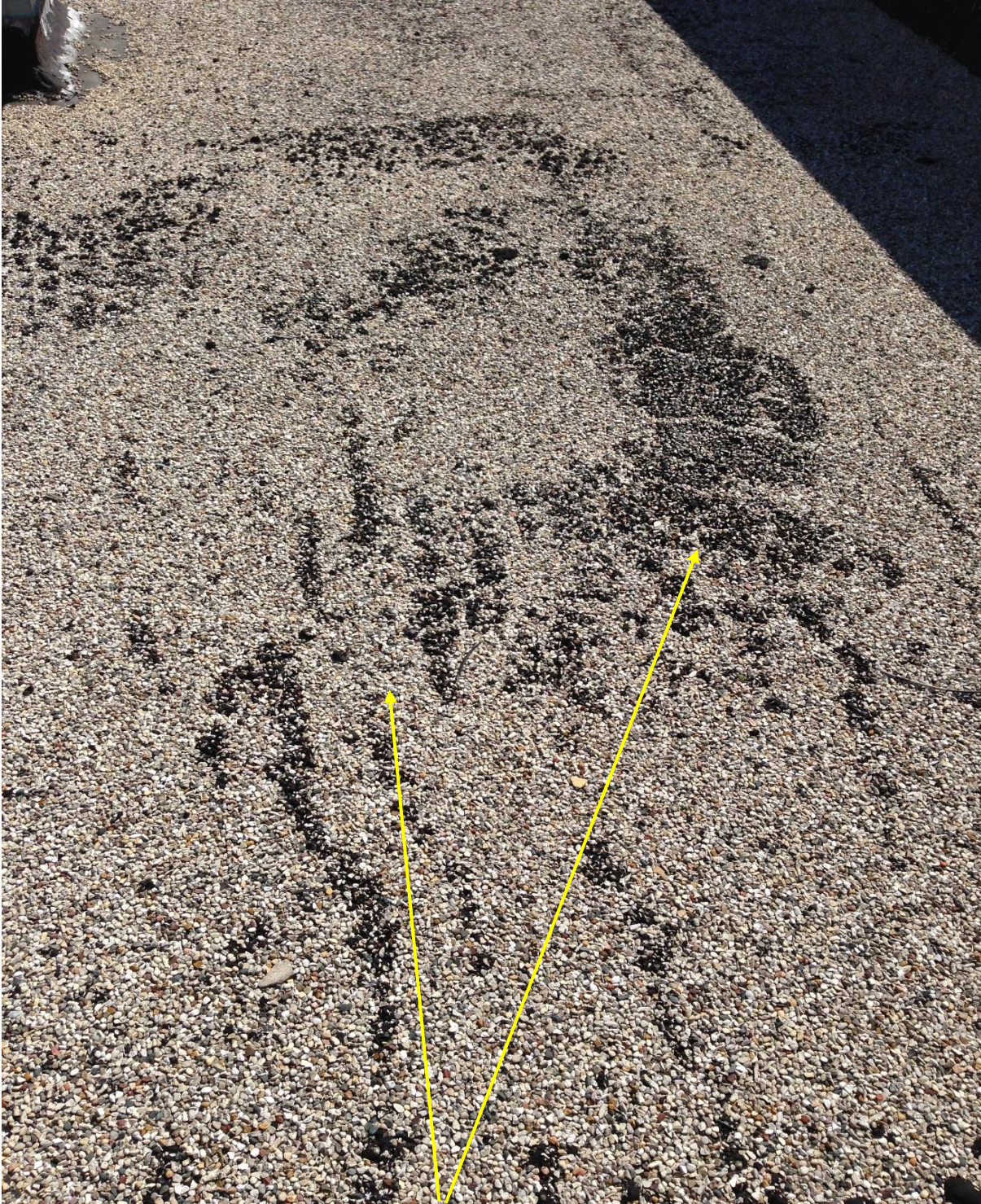
Deteriorated roofing
