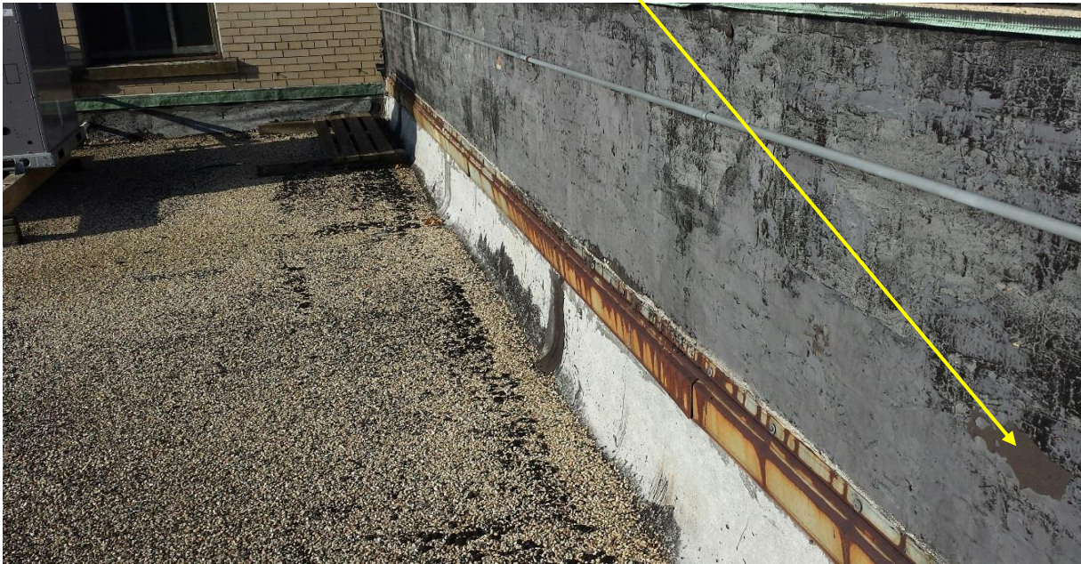
Deteriorated waterproofing
