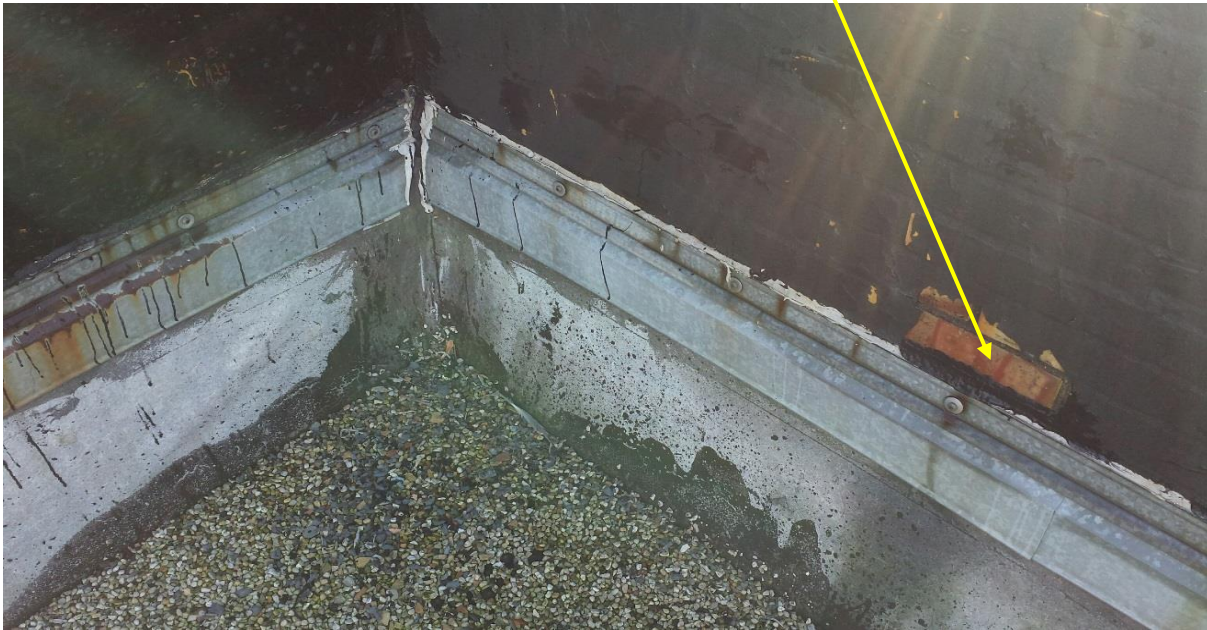
Deteriorated waterproofing
