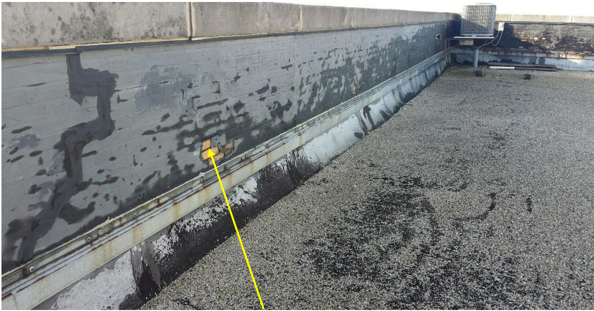
Deteriorated waterproofing
