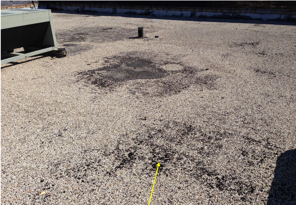
Deteriorated roofing
