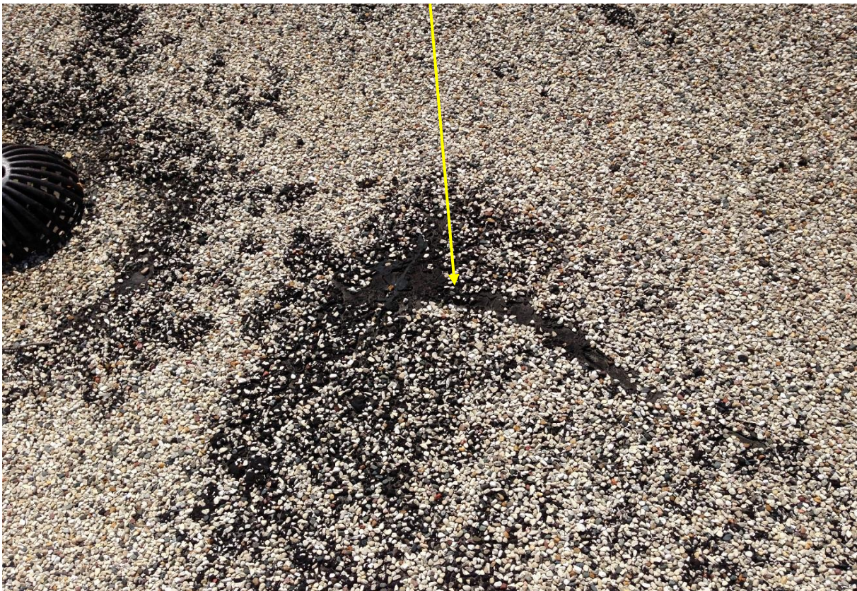
Deteriorated roofing
