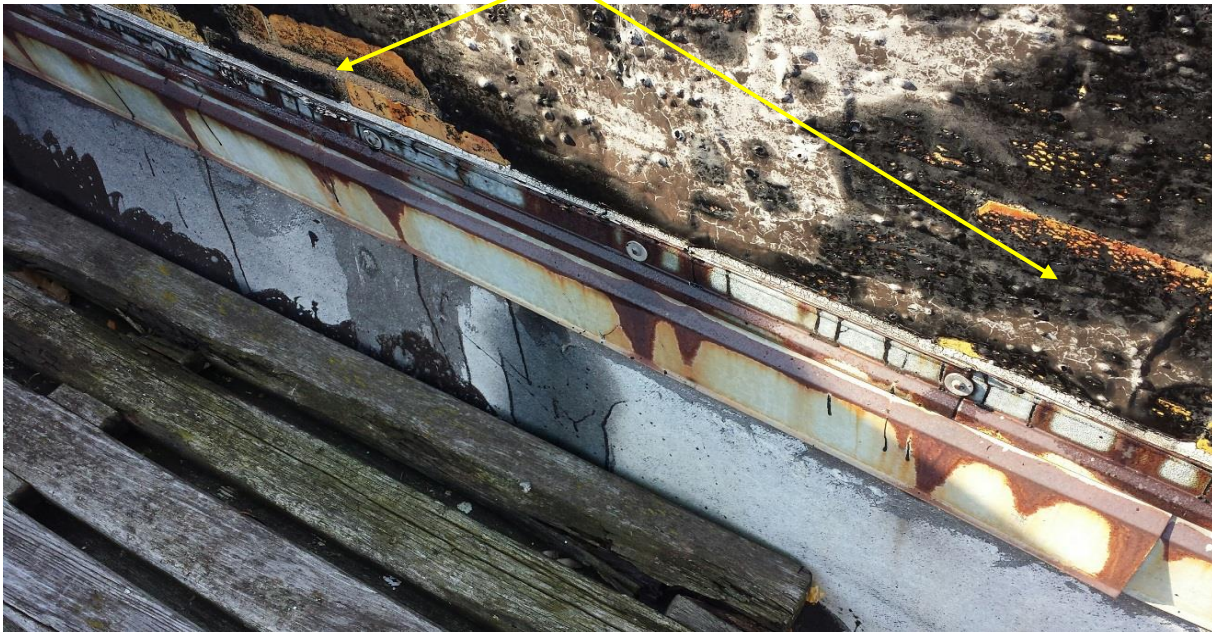
Deteriorated waterproofing
