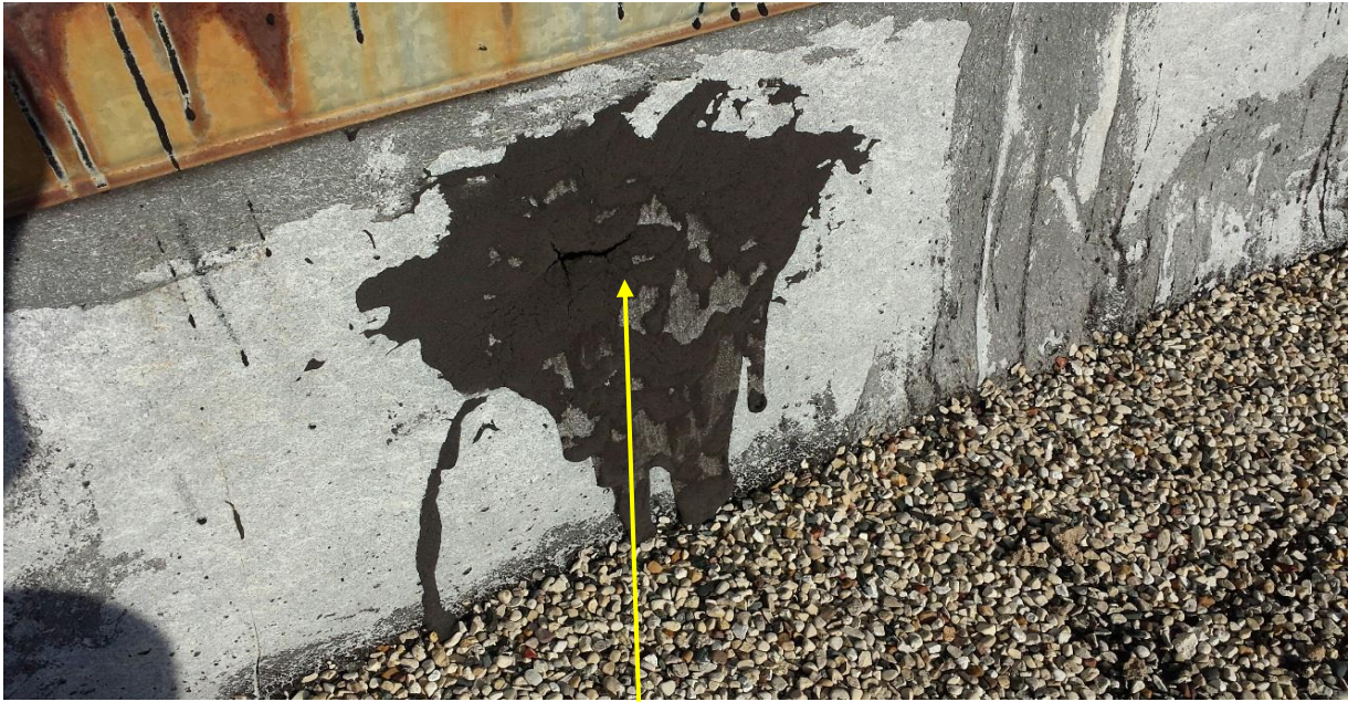
Deteriorated roofing
