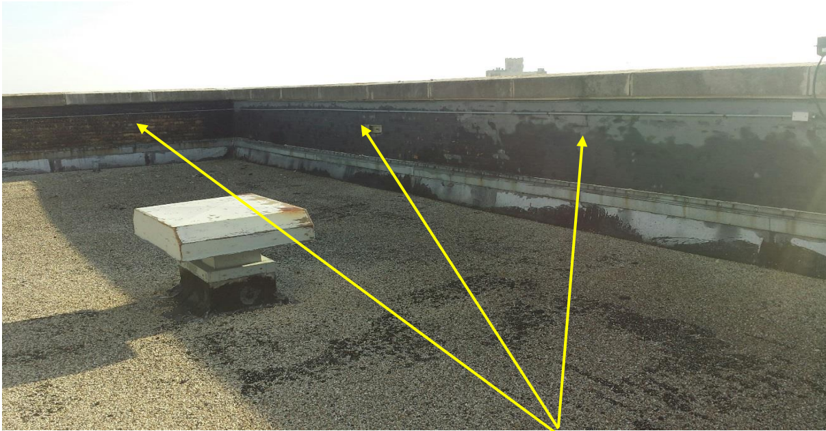
Deteriorated waterproofing
