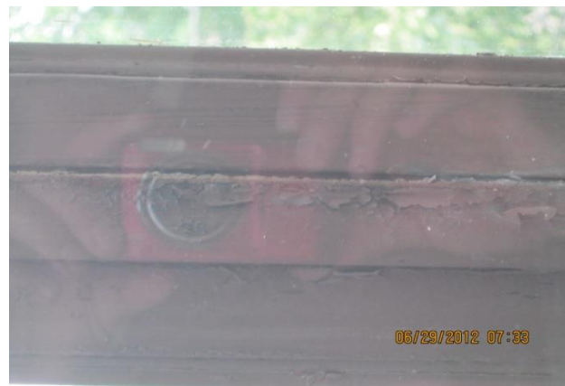
Interior framing corrosion
