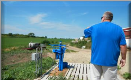
second pumping system to filter area
