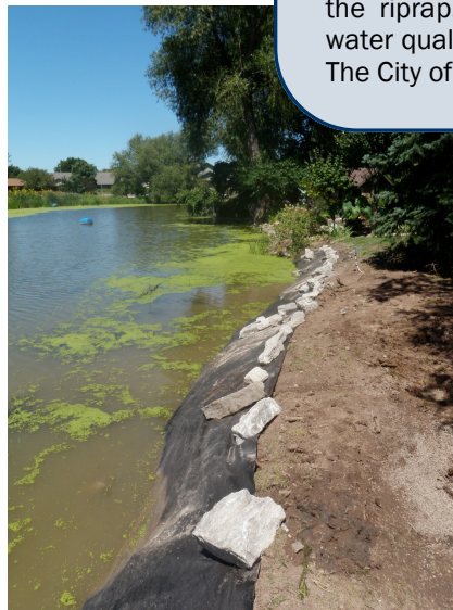
banks re-shaped and geotextile installed before placement of stone
