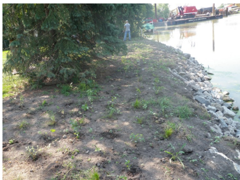
riprap installed with topsoil placed over the top of riprap; native plantings installed on top of riprap and in the uplands
