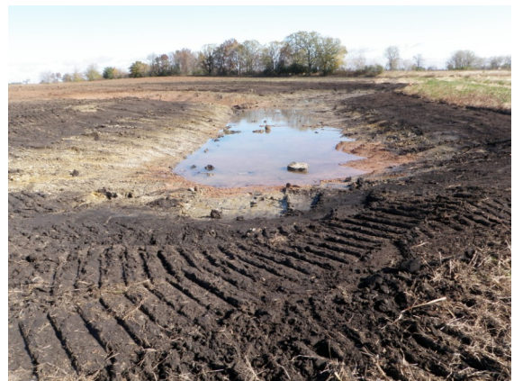
completed wetland scrape
