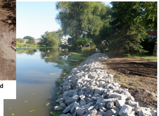
riprap installed along streambank
