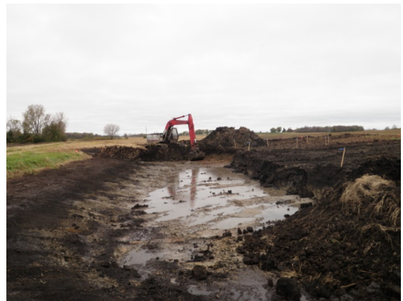
construction of wetland scrape
