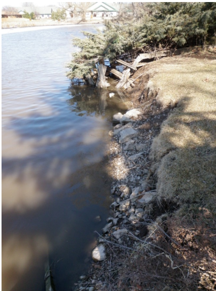
severe streambank erosion
