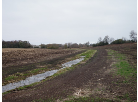
re-grading of grassed waterway
