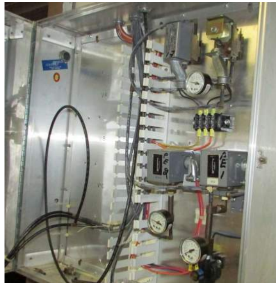
Human Services Center – Oshkosh – Pneumatic Panel
