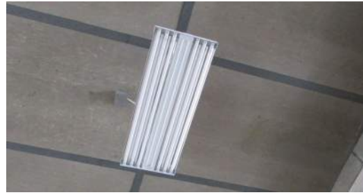
Wittman Field – Basler East Hanger – T8 Lamp Fixture
