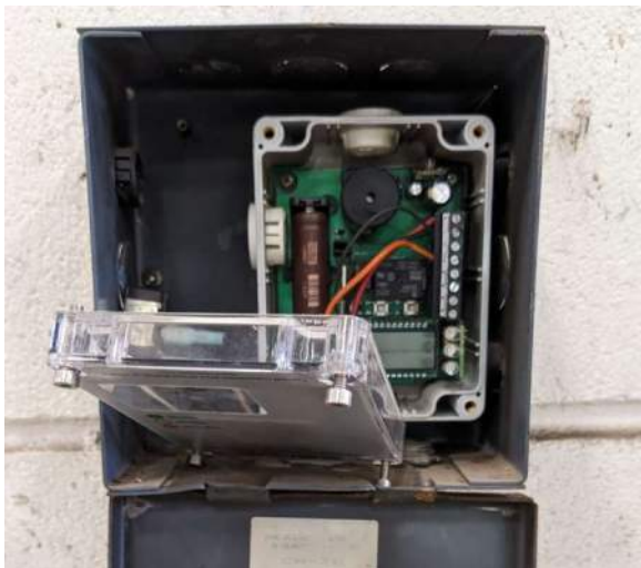
HWY Dept – Storage Garage – Broken CO/NO 2 Sensor
