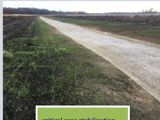
critical area stabilization
