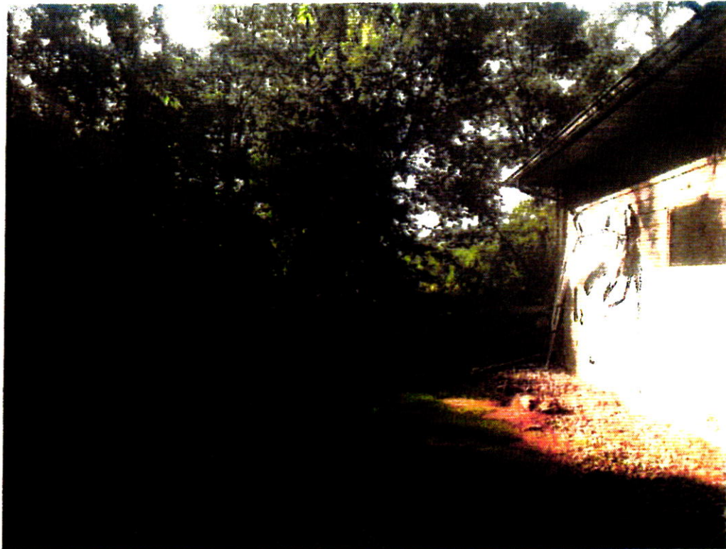
View of Northeast Side of Garage, Looking Southeast
