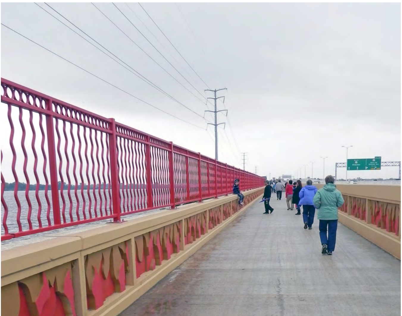
The Fire Bridge on the Tribal Heritage Crossing provides a safe crossing of Lake Butte des Morts for people bicycling and walking.
