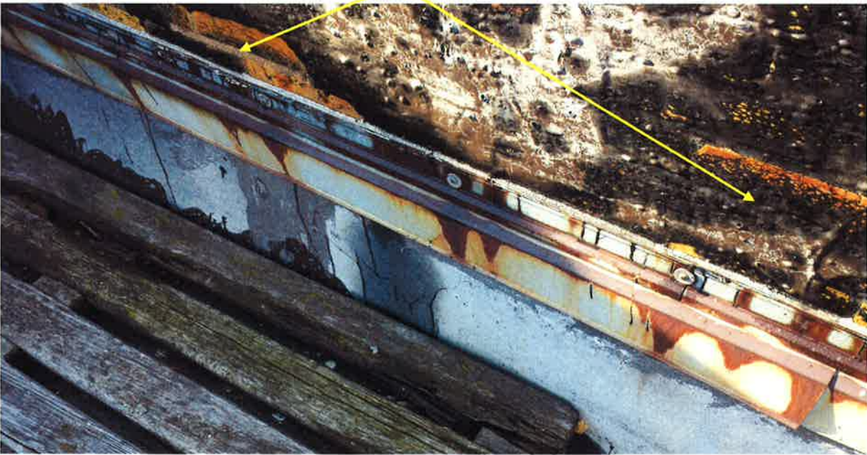
Deteriorated waterproofing
