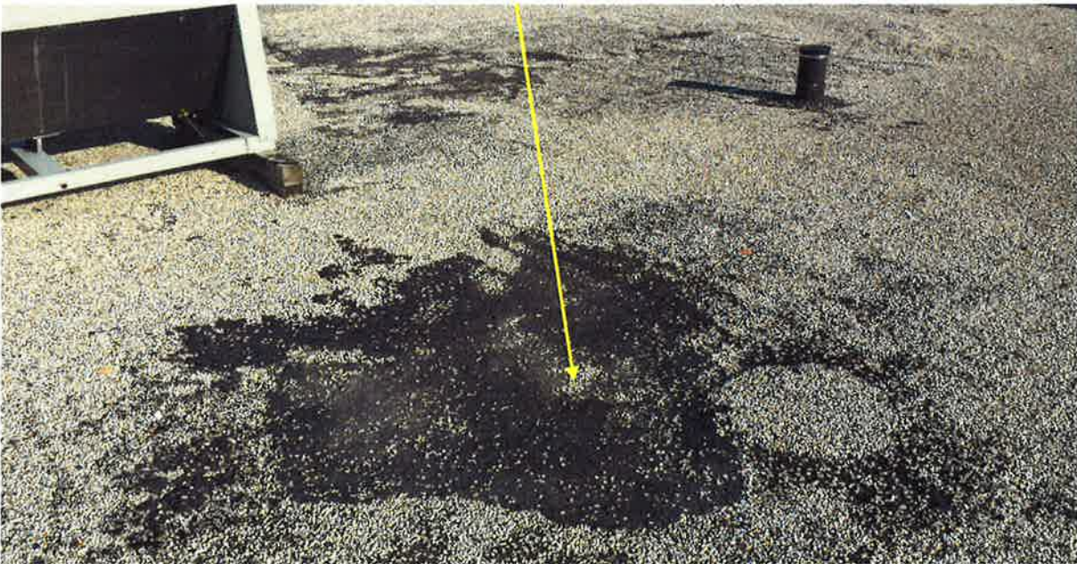
Deteriorated roofing
