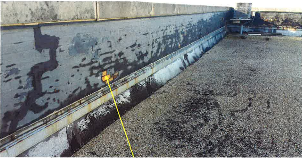
Deteriorated waterproofing
