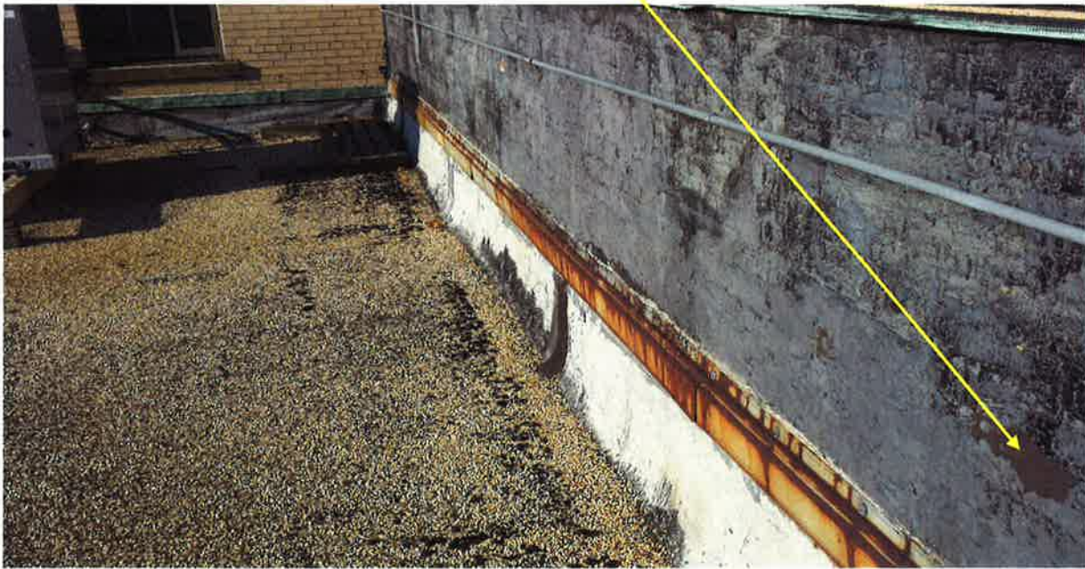
Deteriorated waterproofing
