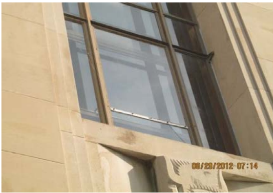
Deteriorated window framing replaced
