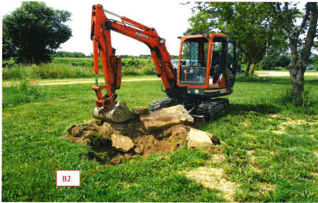
PHOTO 6: VIEW OF TYPICAL FILL MATERIAL FOUND AT B1 & B2
