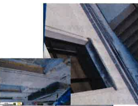
8. EXAMPLES OF MASONRY AND WINDOW SILL NEEDING CHEMICAL CLEANING
