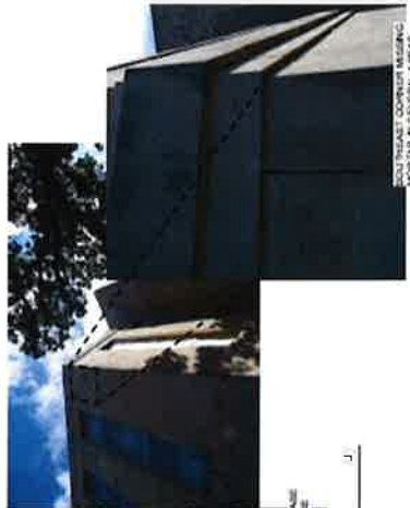
7. EXAMPLES OF REPOINTING 100% AT UPPER BASE AROUND THE COURTHOUSE
