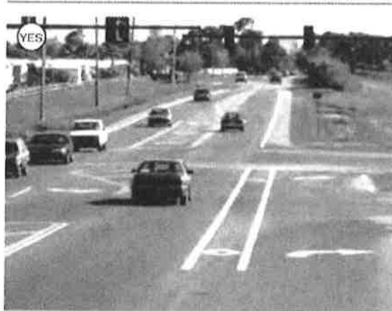
Figure 3-37. This intersection features a bicycle lane to the left of a right-turn lane. Note how it lines up with the bicycle lane on the far side of the intersection.
