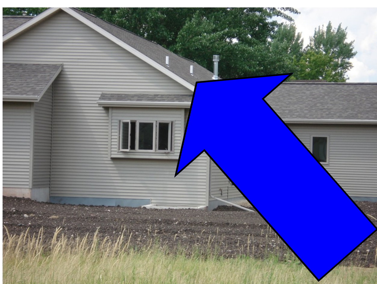
A radon mitigation system is barely visible from the exterior of the house.
