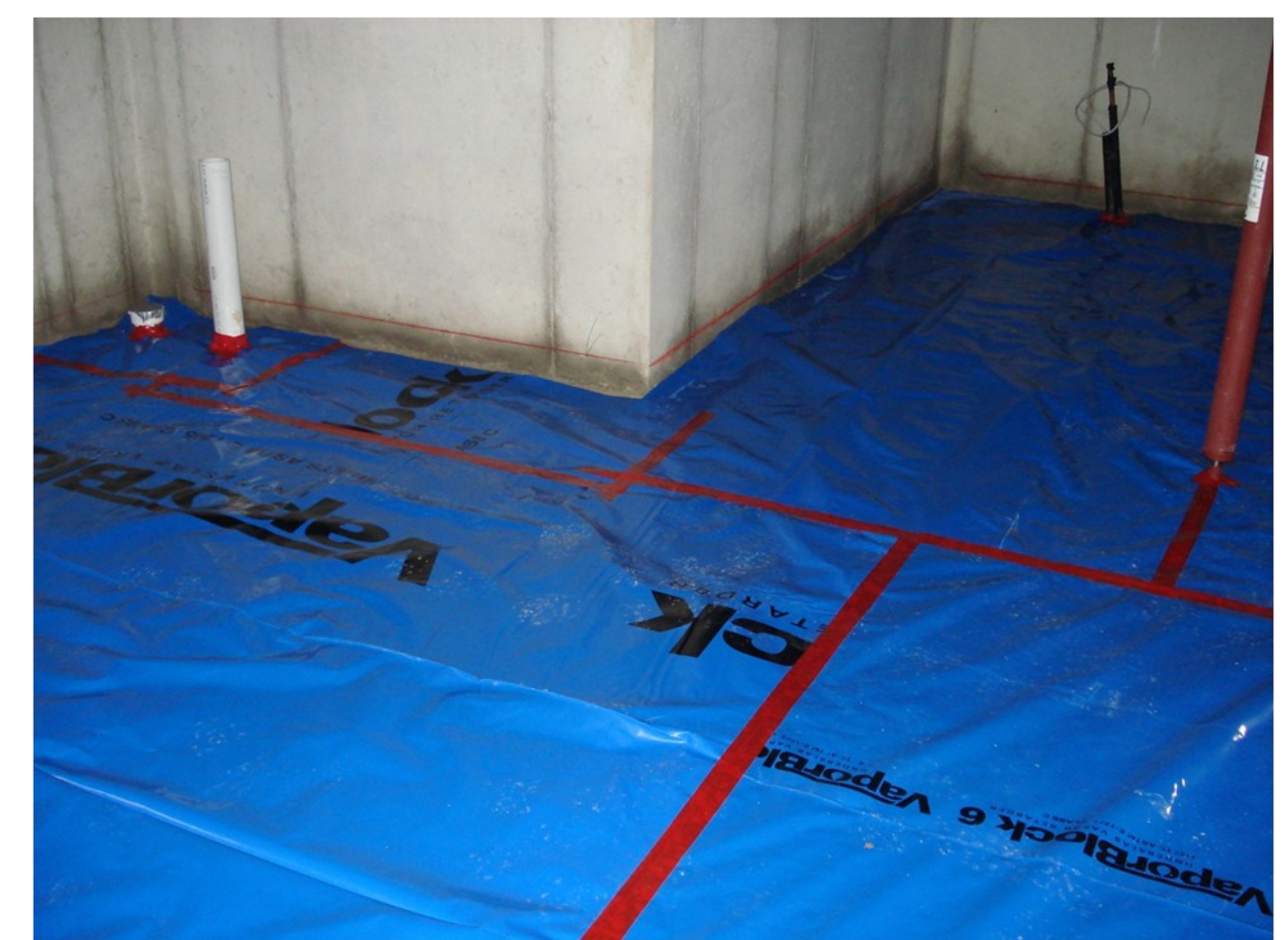
Plastic sheeting over the gravel should be 6 mil in thickness, overlapped by 12 inches, and taped at the seams.
