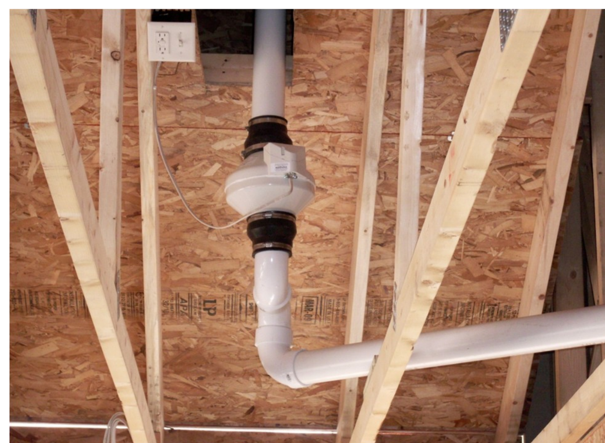
If the pipe by itself does not lower radon levels sufficiently, a fan is installed in the attic to pull radon from below the foundation and out the roof.
