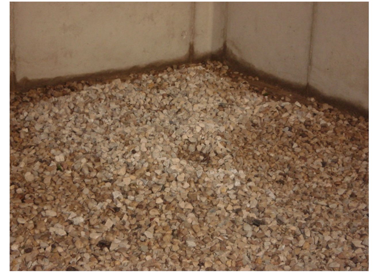
A 4-inch layer of \frac{1}{2} " – \frac{3}{4} " gravel forms a gas permeable layer so radon can be collected below the concrete slab.
