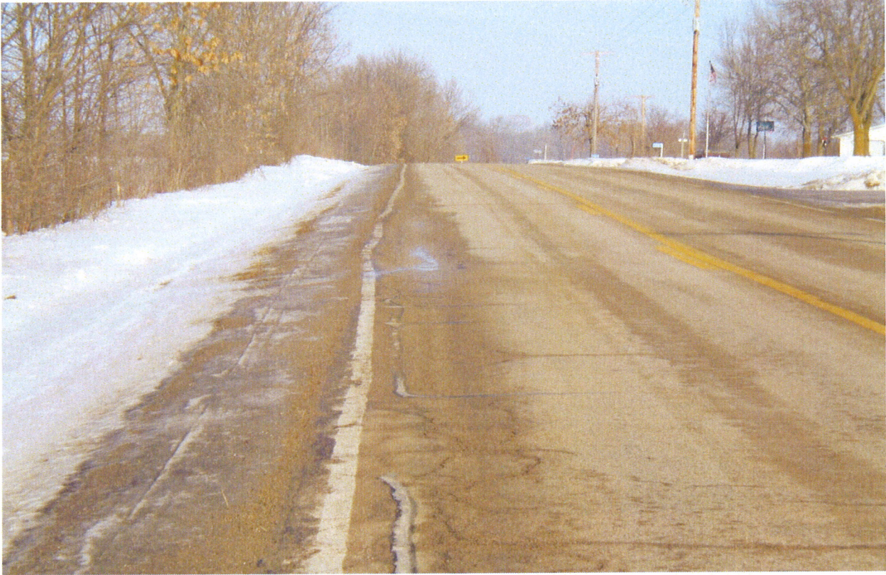
Rutting – *note shoving of edgeline
