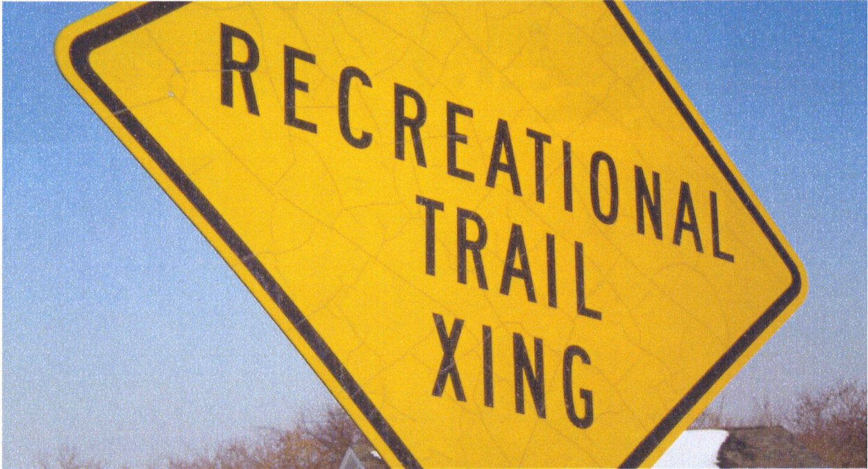
Cracked & faded sheeting. Engineer grade sheeting non-compliant with MUTCD after year 2014
