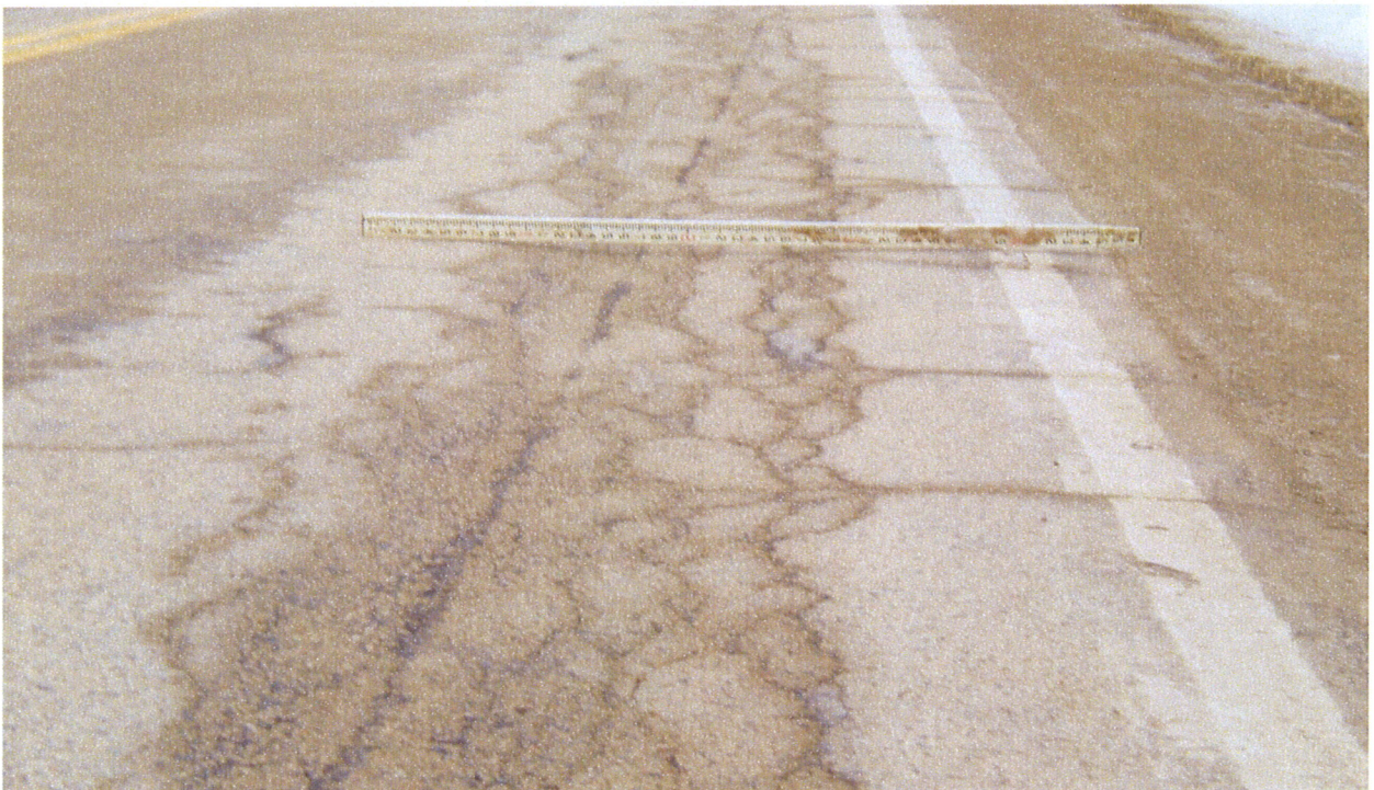
Load cracking and rutting in wheel path
