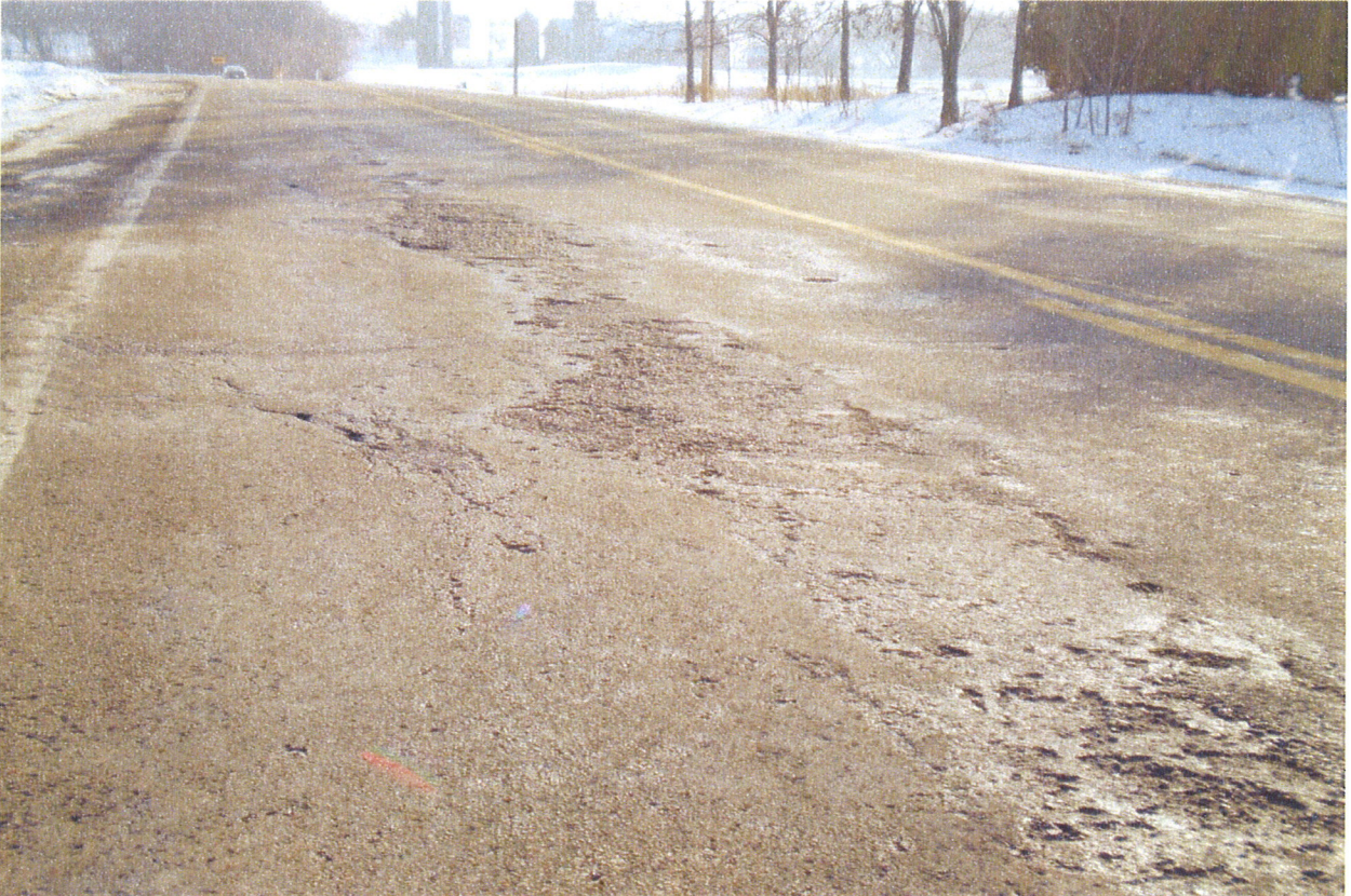
Chipseal slipping - leading to rutting and surface raveling
