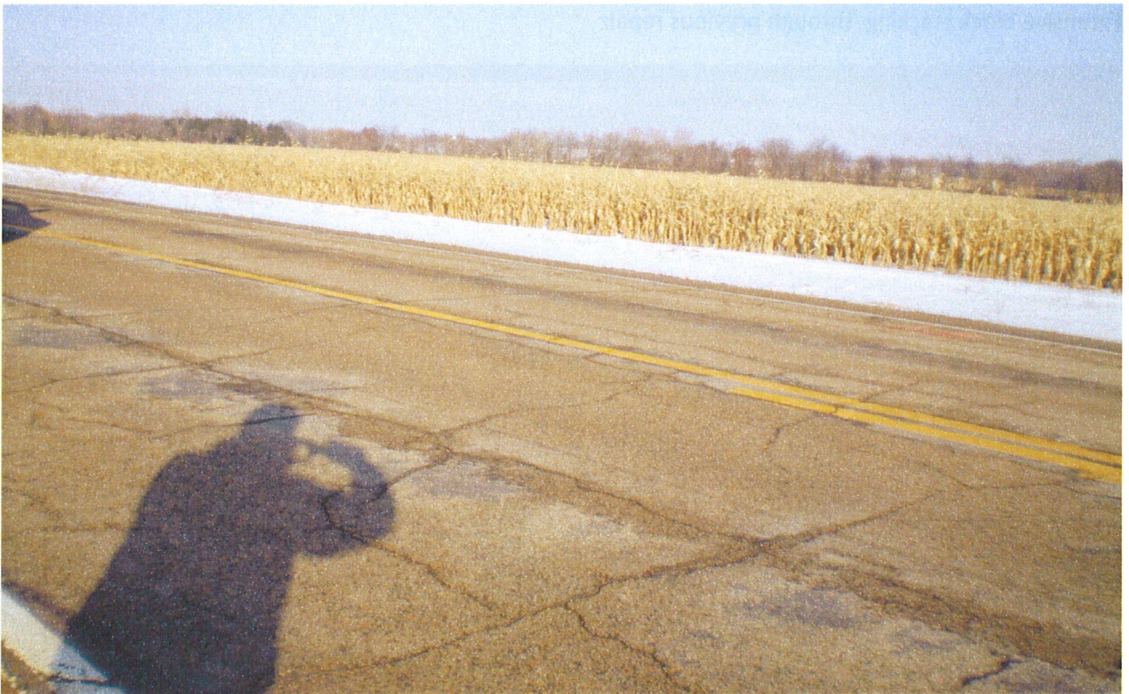
Block cracking
