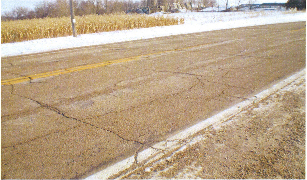
Block cracking
