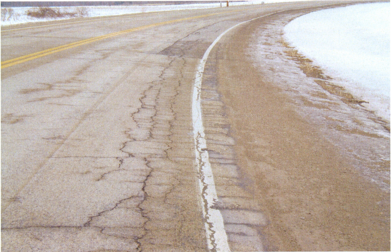
Extensive block cracking through previous repair
