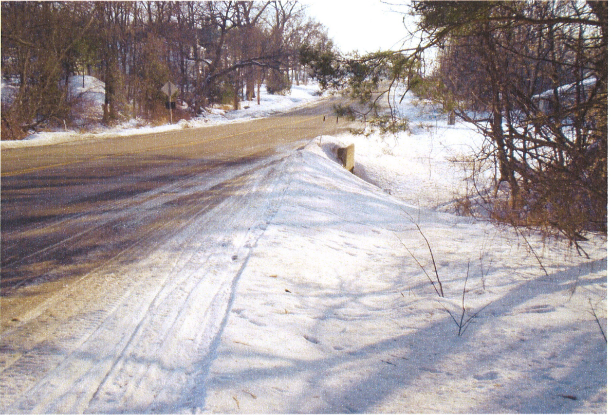
Beam guard needed at box culvert endwall
