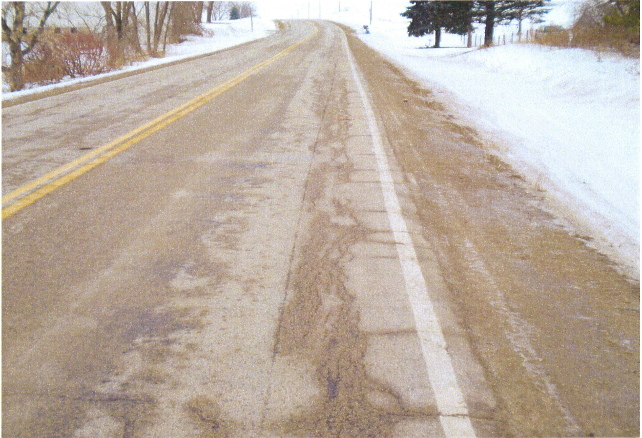
Load cracking and rutting in wheel path
