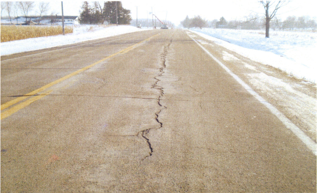
Longitudinal cracks breaking down
