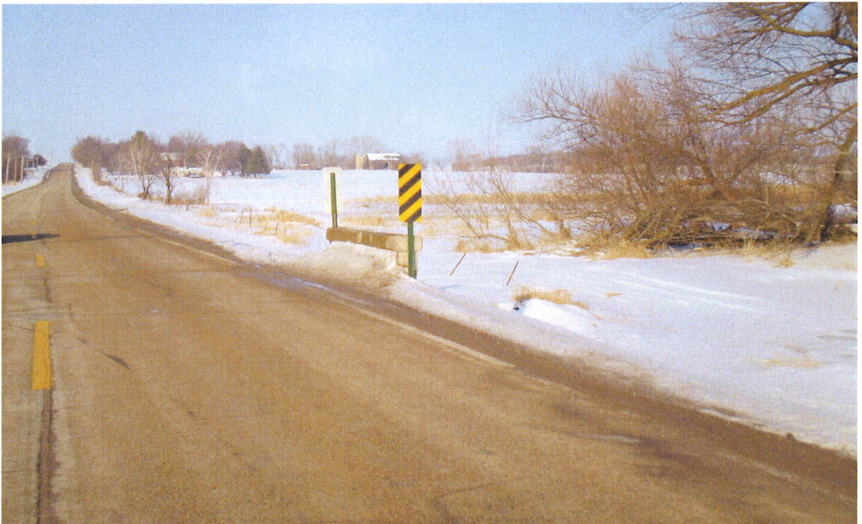
Beam guard needed at parapet walls
