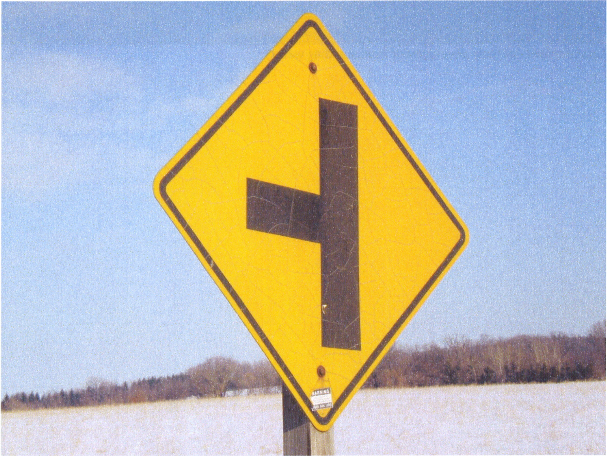
Cracked & faded sheeting. Engineer grade sheeting non-compliant with MUTCD after year 2014
