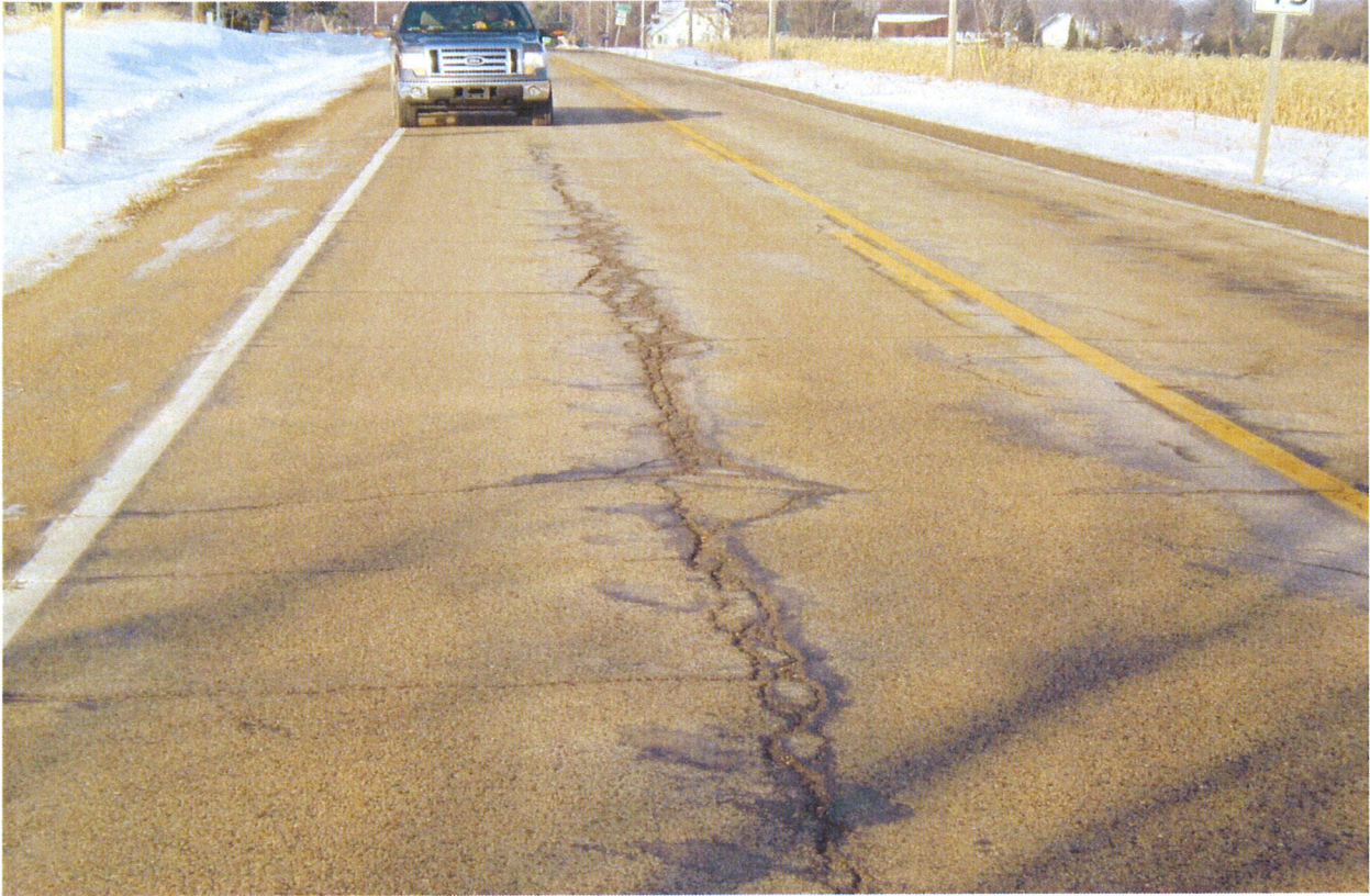
Longitudinal cracks breaking down
