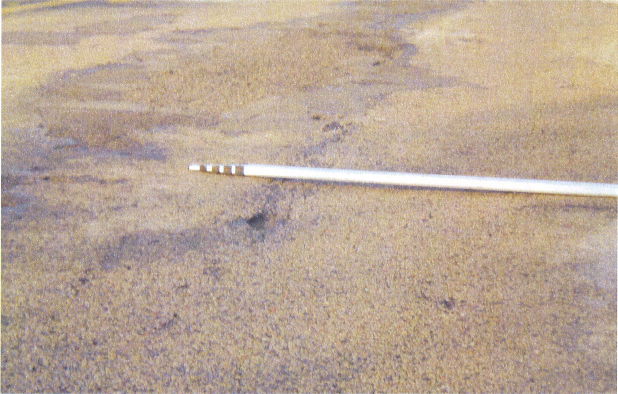
Chipseal slipping - leading to rutting and surface raveling
