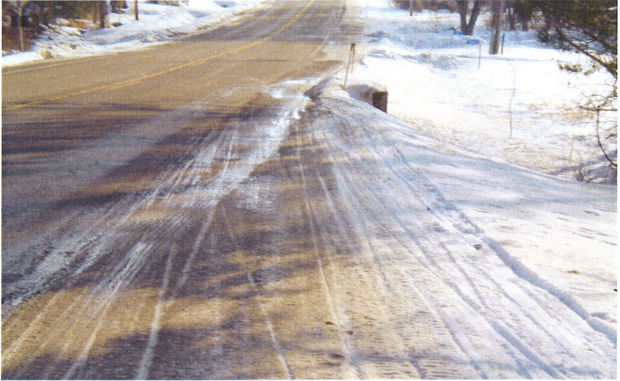
Beam guard needed at box culvert endwall
