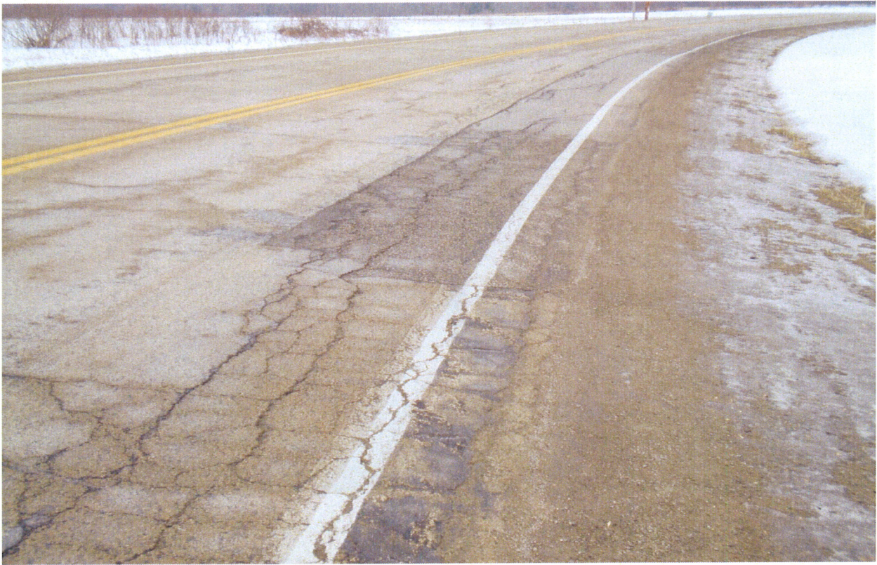
Extensive block cracking through previous repair
