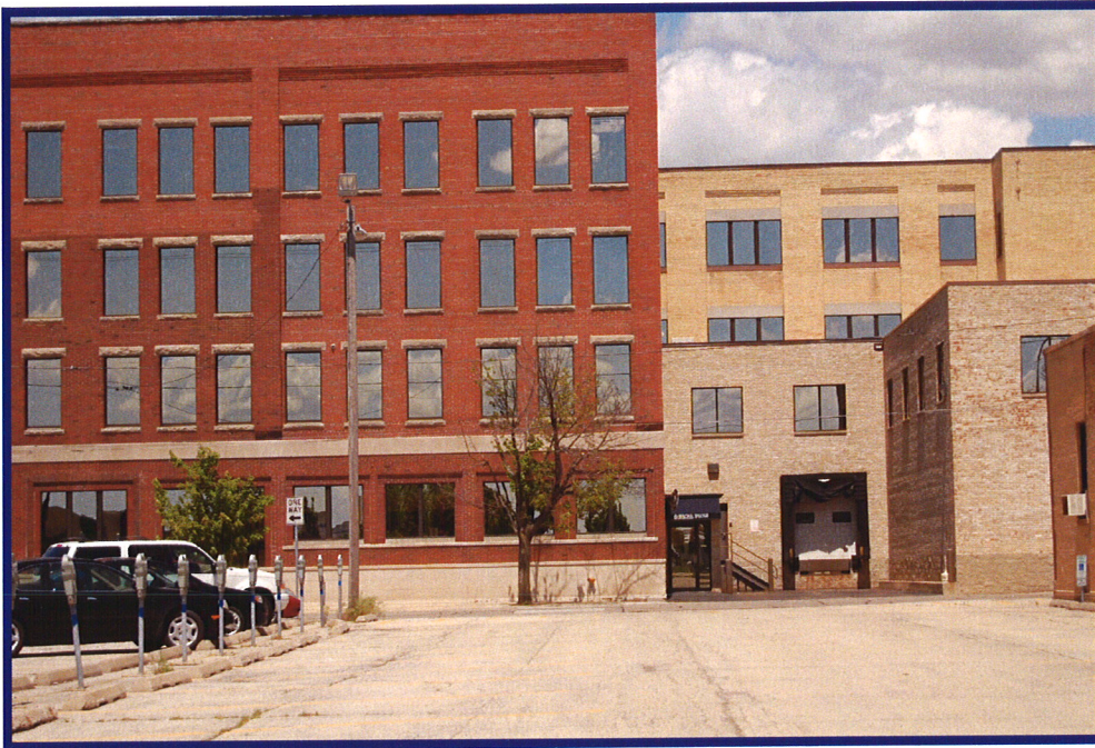
Exterior of warehouse (loading dock and 2-story building right of the main building)
