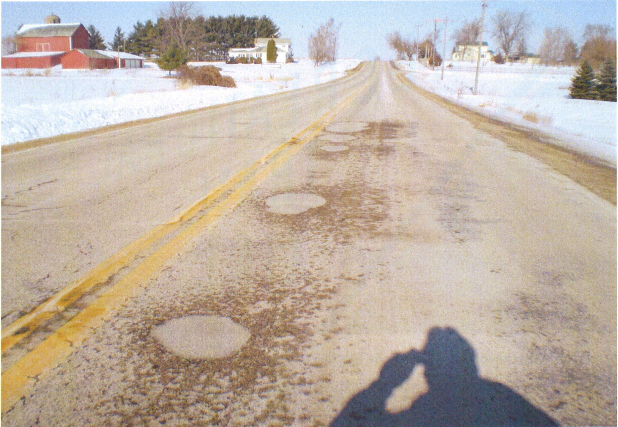
Loss of crown –pothole development from standing water
