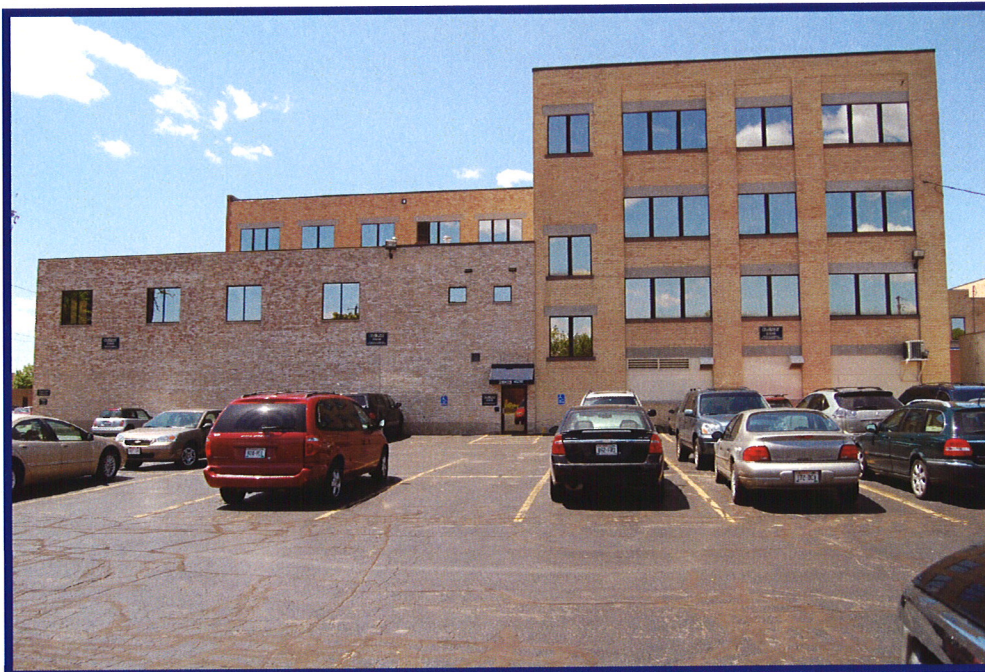
Side view of main building; 128-stall private parking lot with security cameras.
