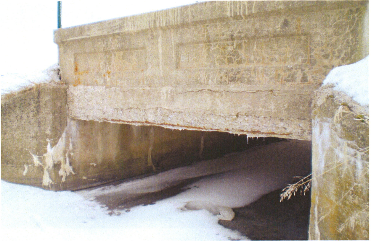
Concrete repair needed
