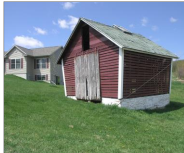
Exhibit 7-1 An example of a rural accessory building
