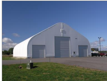
Exhibit 3-5 An example of a polystructure
